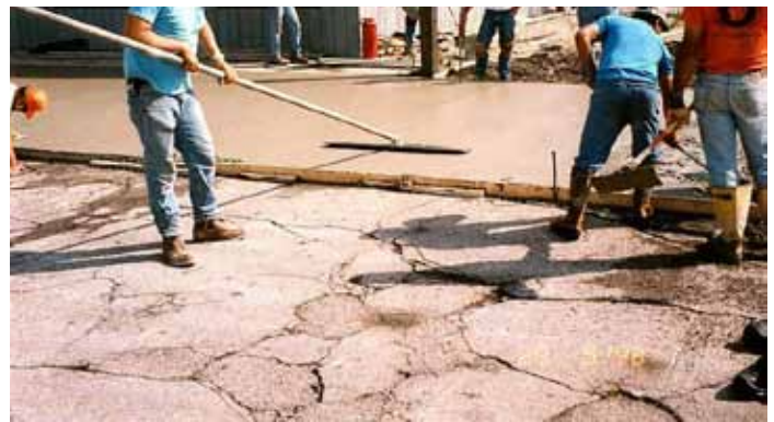
Figure 2. Unbonded concrete overlay (new concrete pavement) being constructed over high-severity distressed asphalt parking lot
