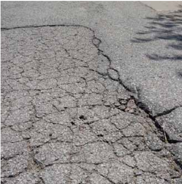
Figure 10b. High-severity alligator cracking
