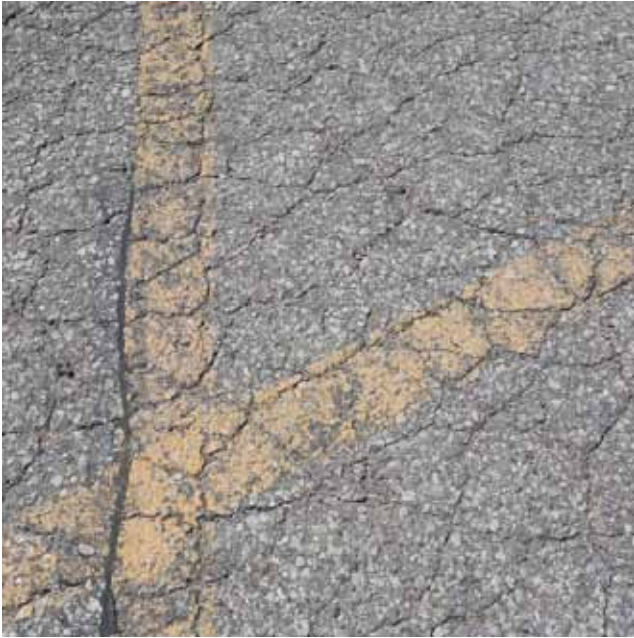
Figure 10a. Low- to medium-severity alligator cracking
