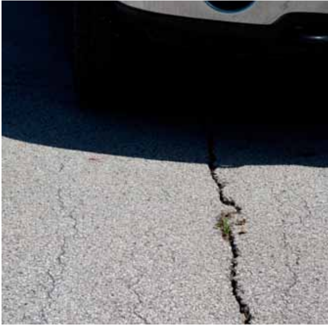
Figure 14a. Low- to medium-severity thermal cracking
