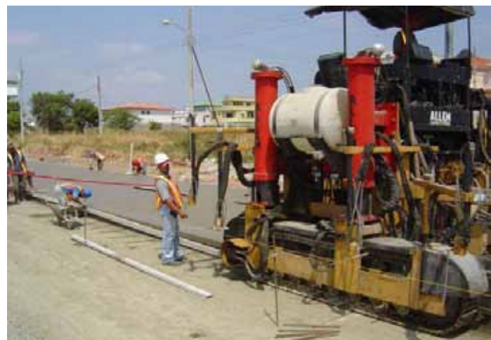
Figure 48. The slipform paver is used for high production paving without using side forms, following a string line or GPS to maintain proper grade and steering; typically used when paving over 50,000 sq ft of pavement per day
