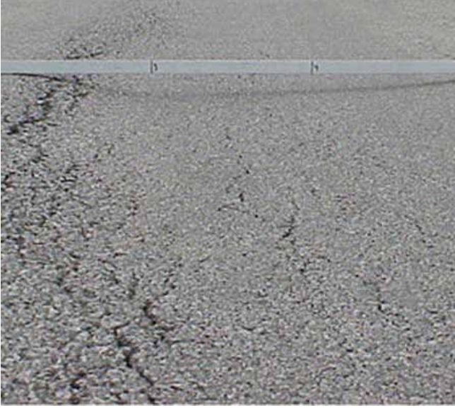
Figure 16a. Low- to medium-severity rutting
