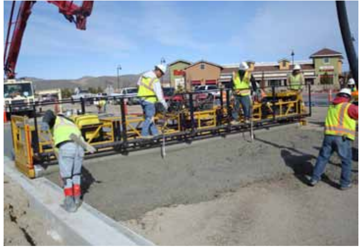
Figure 44. This high production, non-vibrating spinning triple-roller tube paver is used on small, medium, or large projects at paving widths from 10- to 32-ft wide; flat pavements up to 50,000 sq ft/day
