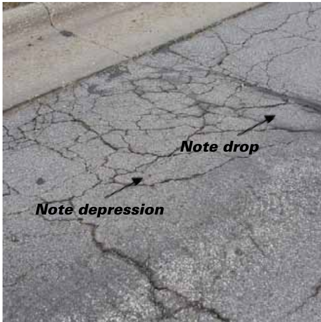
Figure 11b. High-severity block cracking
