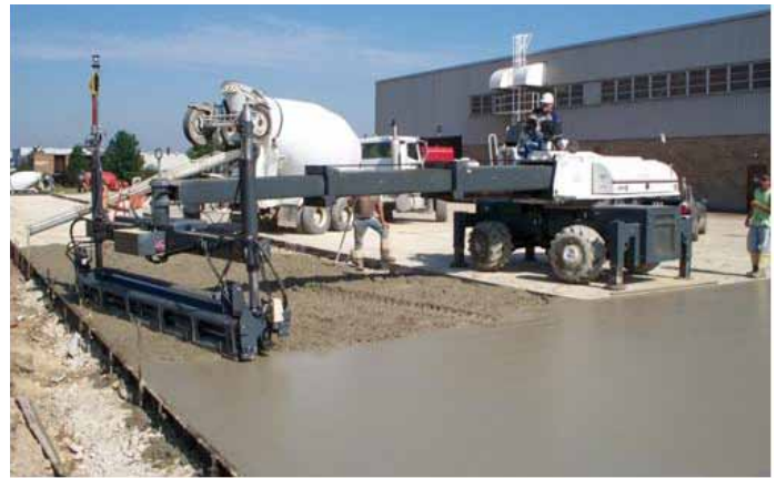
Figure 46. This ride-on boom style laser-guided screed will pave flat, crowned, or inverted pavements with 3D Profile Package installed; typically used when long wide areas of 20,000 to 50,000 sq ft to minimize the amount of time setting forms
