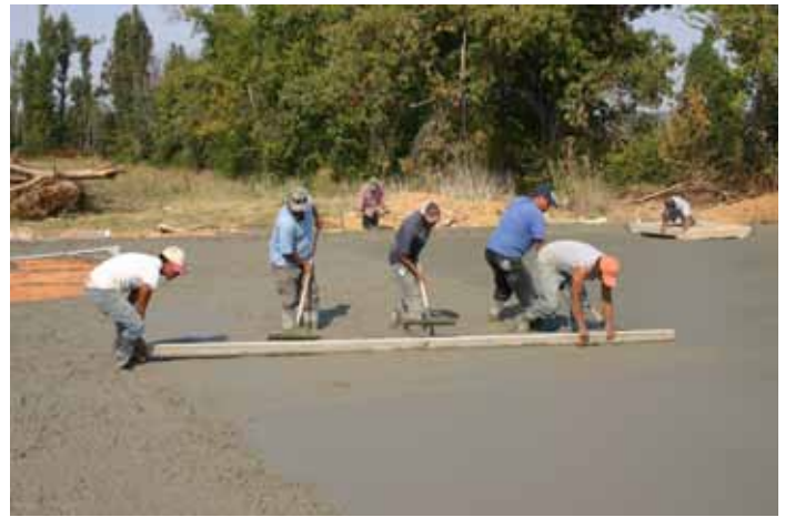
Figure 39. “Striking off” with hand wet screed
