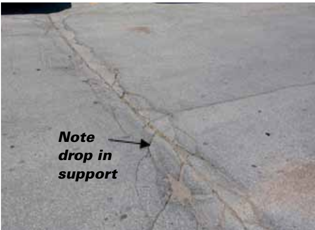
Figure 15c. High-severity random cracking
