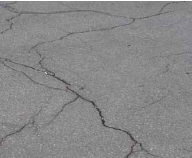
Figure 15b. Low- to medium-severity random cracking
