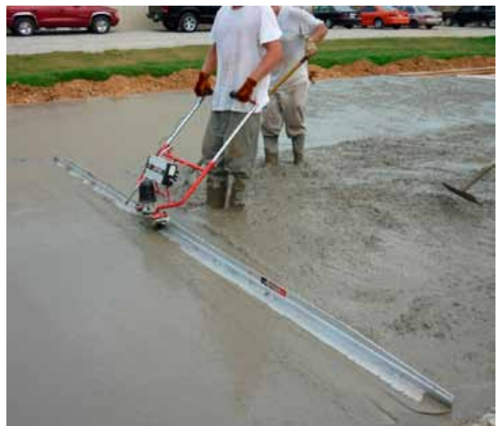
Figure 41. Mechanical vibrating floating screed
