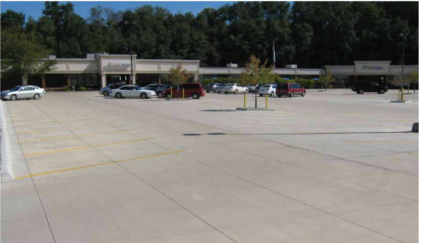
Completed 4-in. bonded concrete overlay of approximately 20-year-old asphalt parking lot pavement with low- to medium-severity distress; Armar commercial center, Marion, IA
