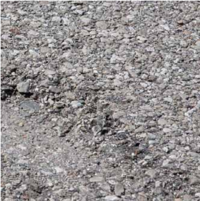
Figure 13b. High-severity raveling
