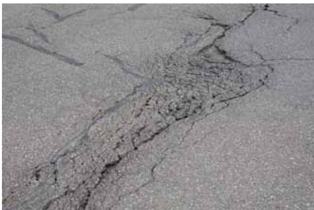
Figure 12a. Low- to medium-severity pothole
