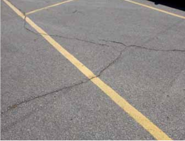
Figure 15a. Low- to medium-severity random cracking
