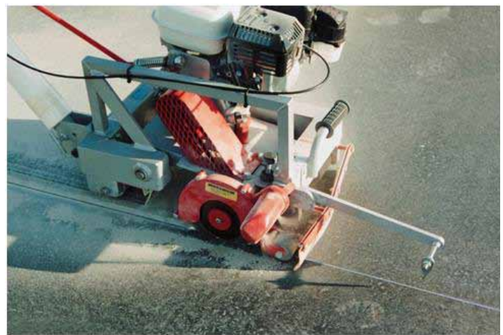
Figure 50. Early-entry saw, which enables sawing within one to two hours of finishing and before final set to minimize random cracking
