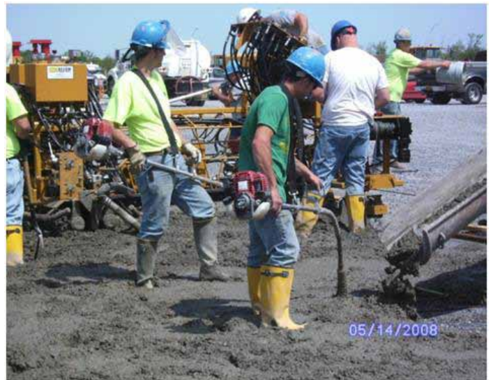
Figure 40. Concrete vibrator
