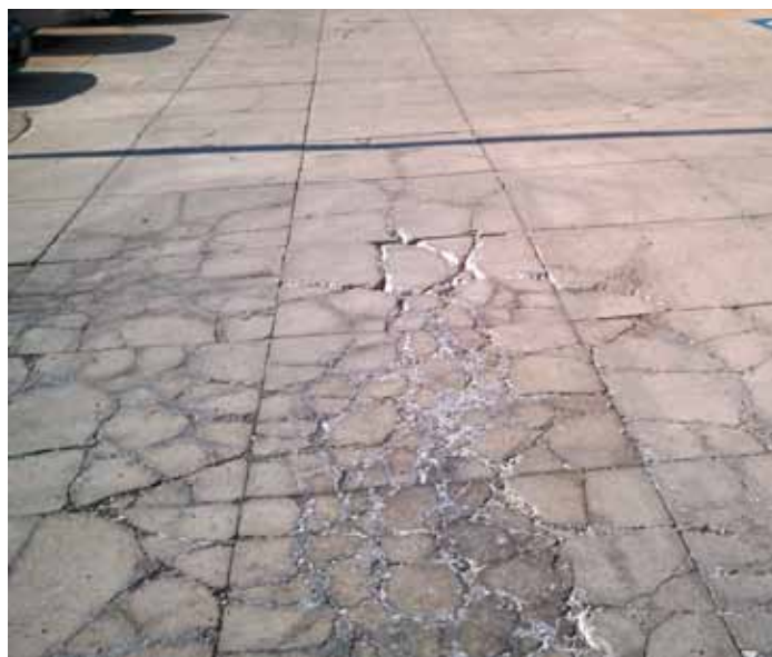
Figure 8. Failure of concrete overlay sections in locations where the existing asphalt pavement surface was entirely removed through milling because of lack of core information
