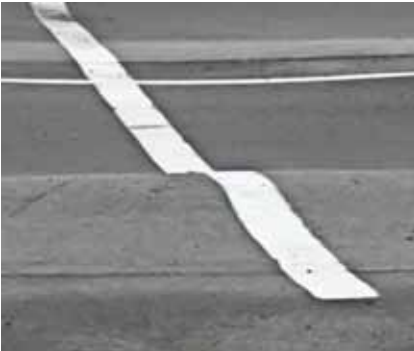
Figure 16b. High-severity rutting
