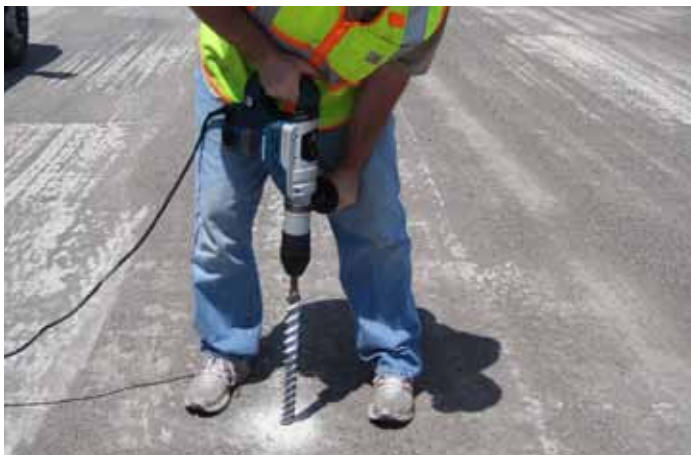
Figure 6. Hammer drilling to check pavement thickness (Photo courtesy of David White, Iowa State University)
