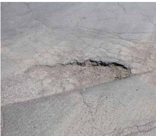
Figure 12b. High-severity pothole
